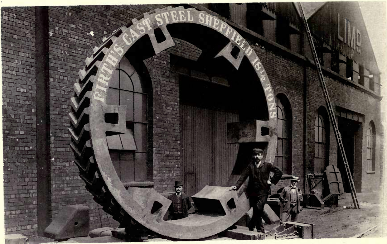
STEEL CASTING, WEIGHT 18\frac{1}{2} TONS.
