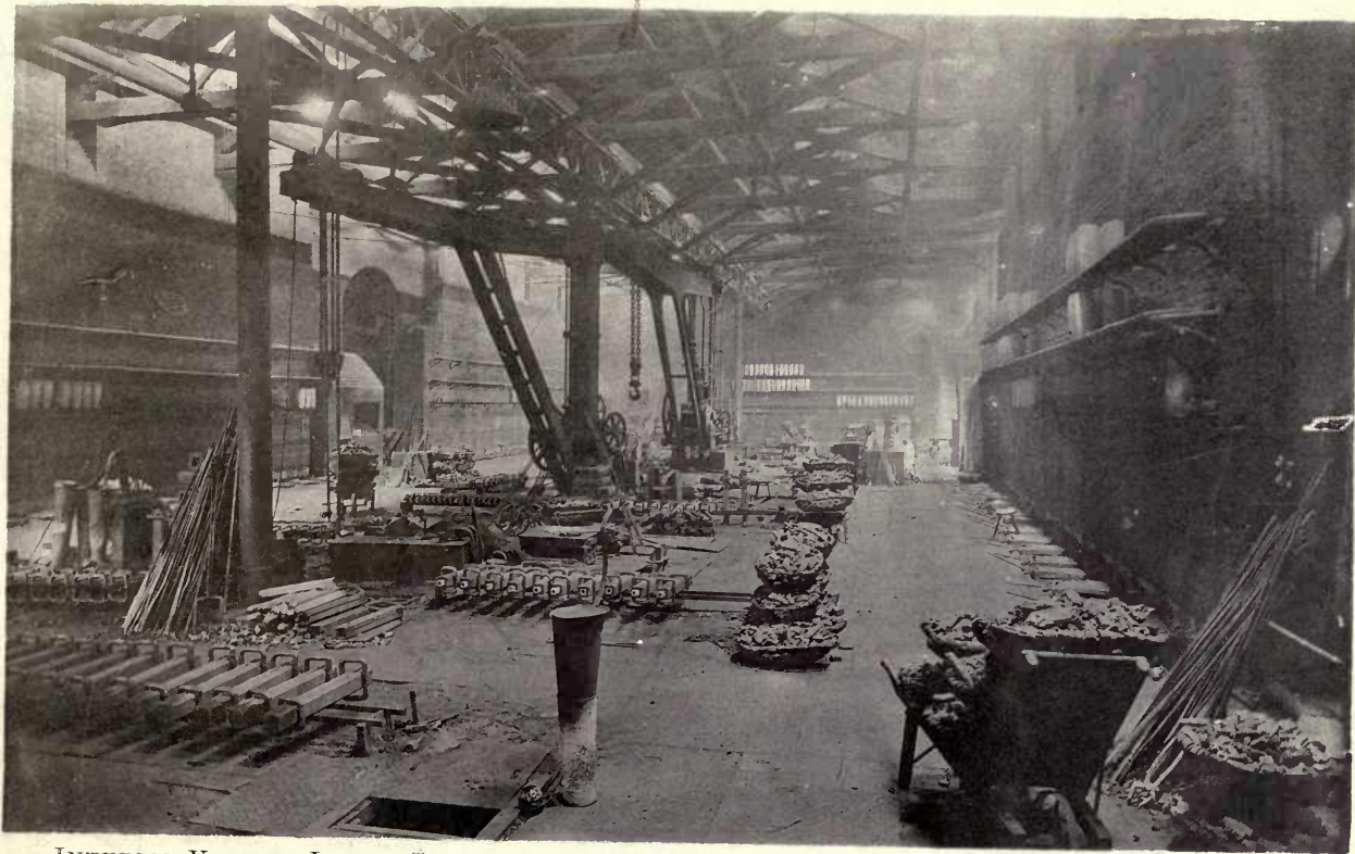
INTERIOR VIEW OF LARGE CRUCIBLE STEEL 100-HOLE MELTING FURNACE AT NORFOLK WORKS. 163 feet long \times 70 feet wide. Area 1,269 square yards.
