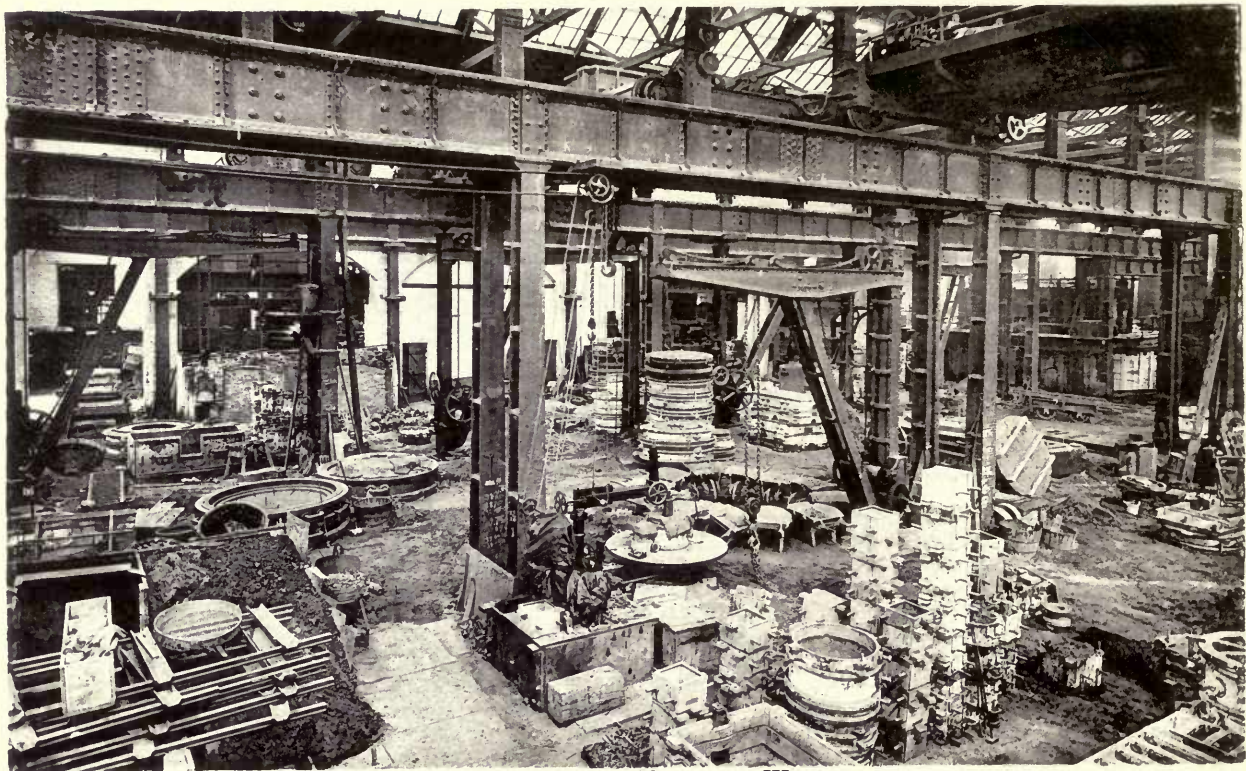
STEEL FOUNDRY, AT NORFOLK WORKS.
