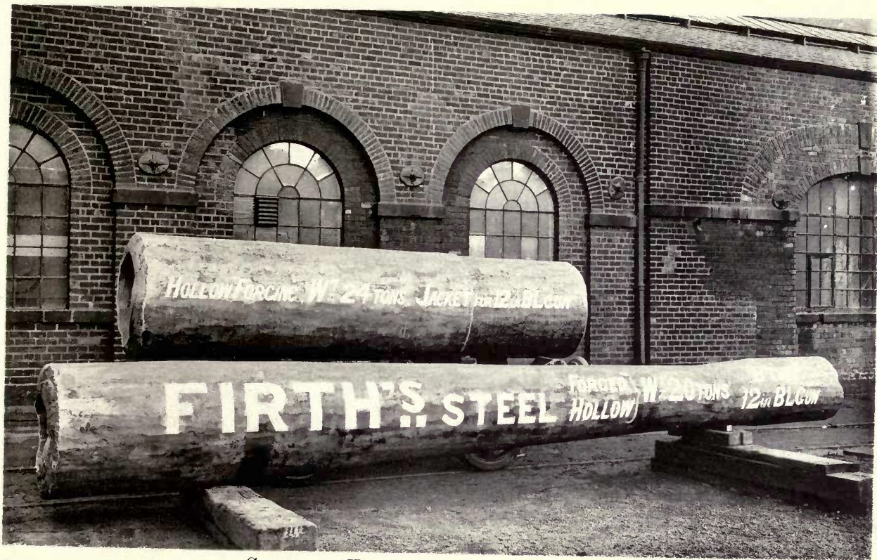
COUPLE OF HOLLOW FORGINGS FOR 12in. B.L. GUN.
