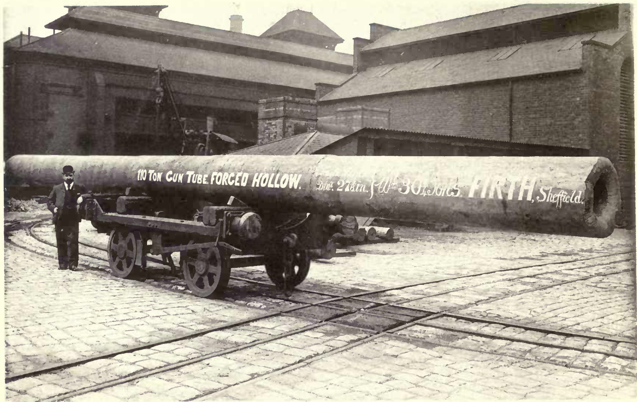
HOLLOW GUN TUBE FORGING.
