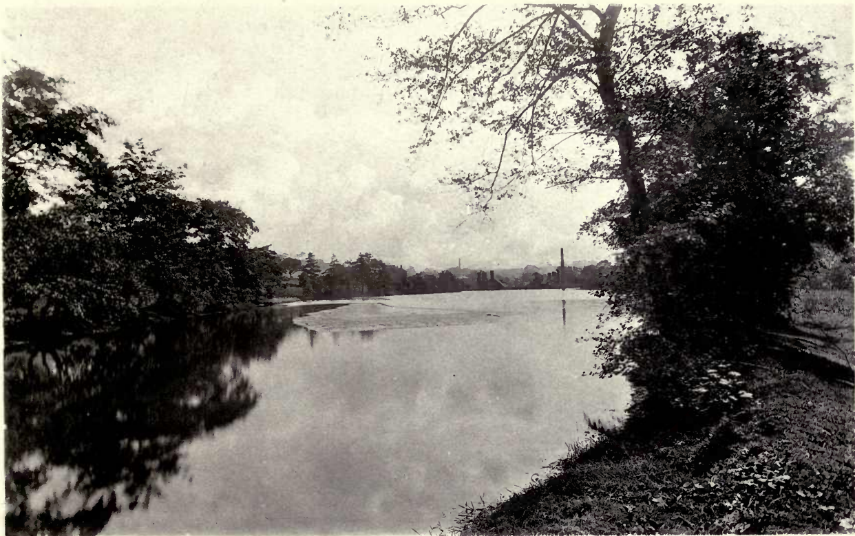
DAM AT CLAY WHEEL FORGES.
