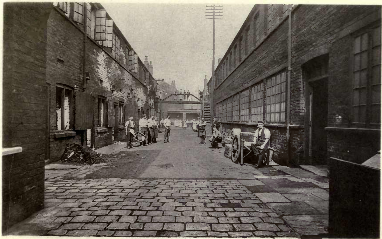
INTERIOR, OLD FILE FACTORY..
