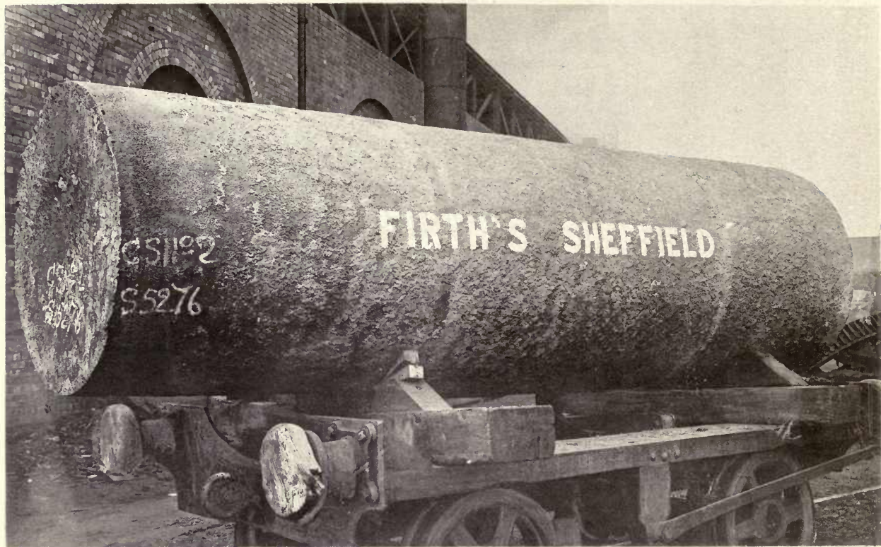
50 TON STEEL INGOT, 53 in. DIAM. \times 180 in. LONG.
